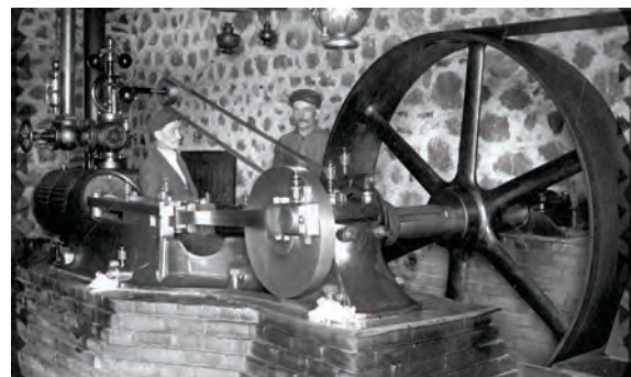
This 60-horse-power steam engine acquired from Frogner Bros., installed at the Iola Mills in late 1898, providing power for their grist and sawmills, was housed in a stone engine house built between the two mills. The walls of this structure still stand between the mill and the dam.
