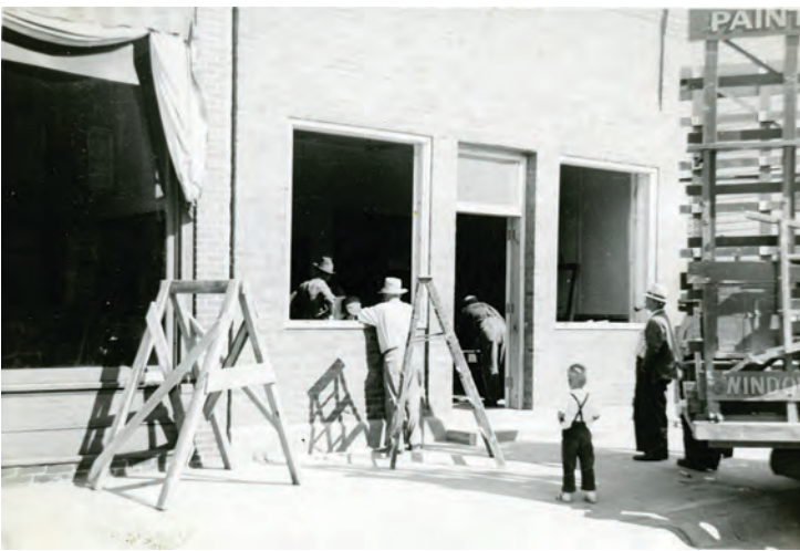
Finishing Touches, Spring 2026
