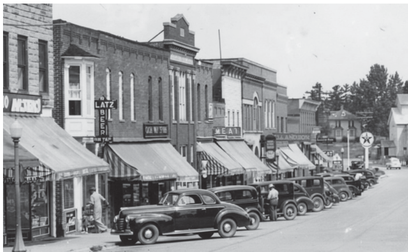
This view of the west side of the business block of North Main Street, from State Street to Depot Street, starts with the Graystone Building and dates from the 1940s.
